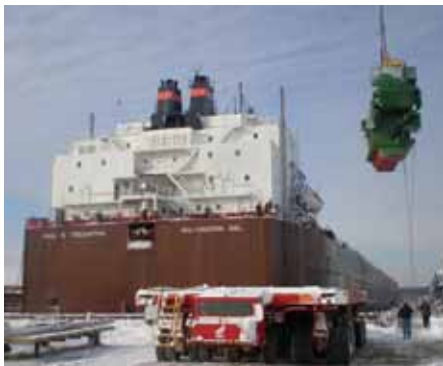
Above and center below: Setting the starboard MAK diesel, December 2009.
